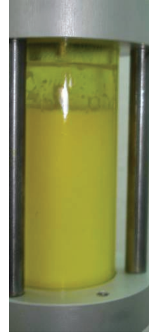
Insufficiently mixed oil and refrigerant.
